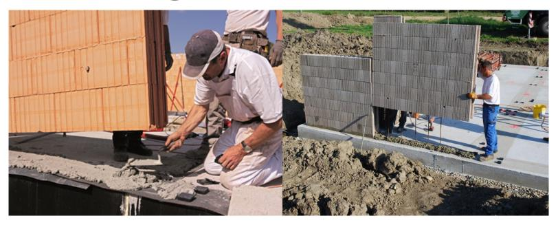
The wall elements are set into a fresh mortar bed.
