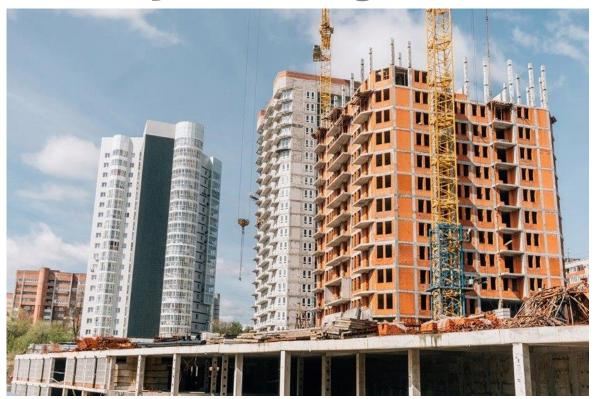
Apartment complex: prefab walls made of aerated concrete blocks and ceramic bricks - redbloc technology
