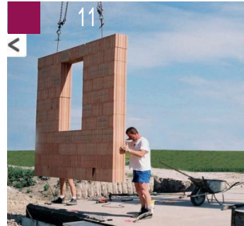
Image 11 • Setting a wall element
