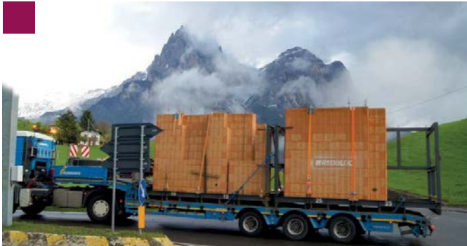
Image 10 • Transport of the finished wall elements to the construction site
